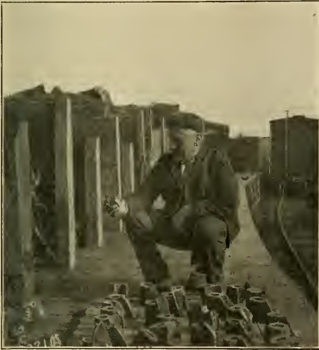
BROKEN KNUCKLES DUE TO LINK SLOTS AND PIN HOLES.
